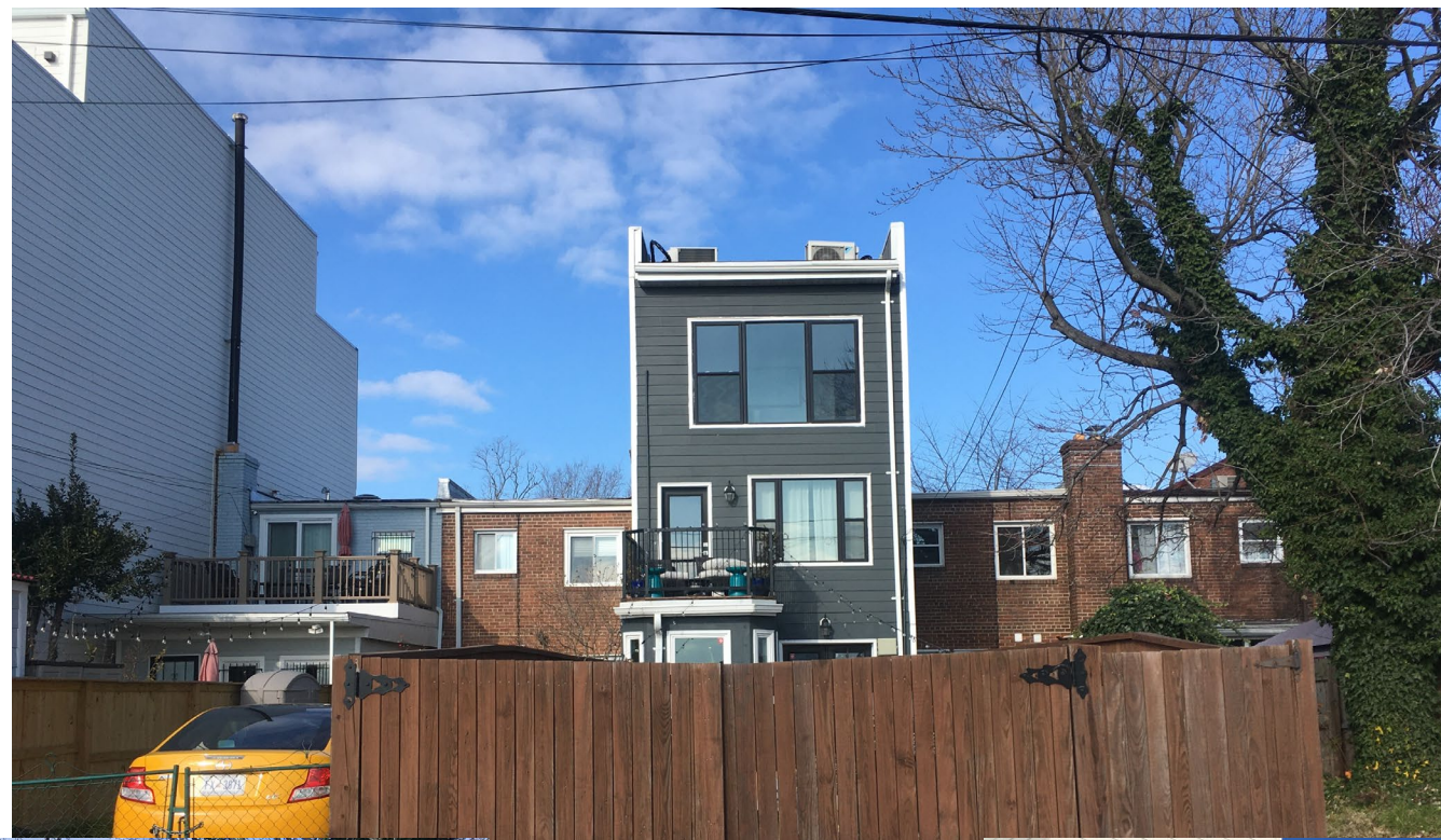
View from Alley (L Street SE) looking North
